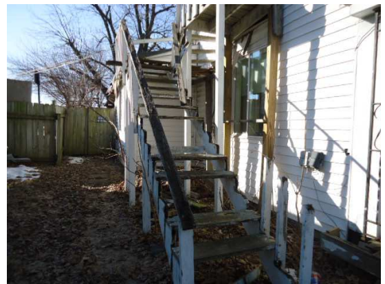
Stairway to Unit 2
